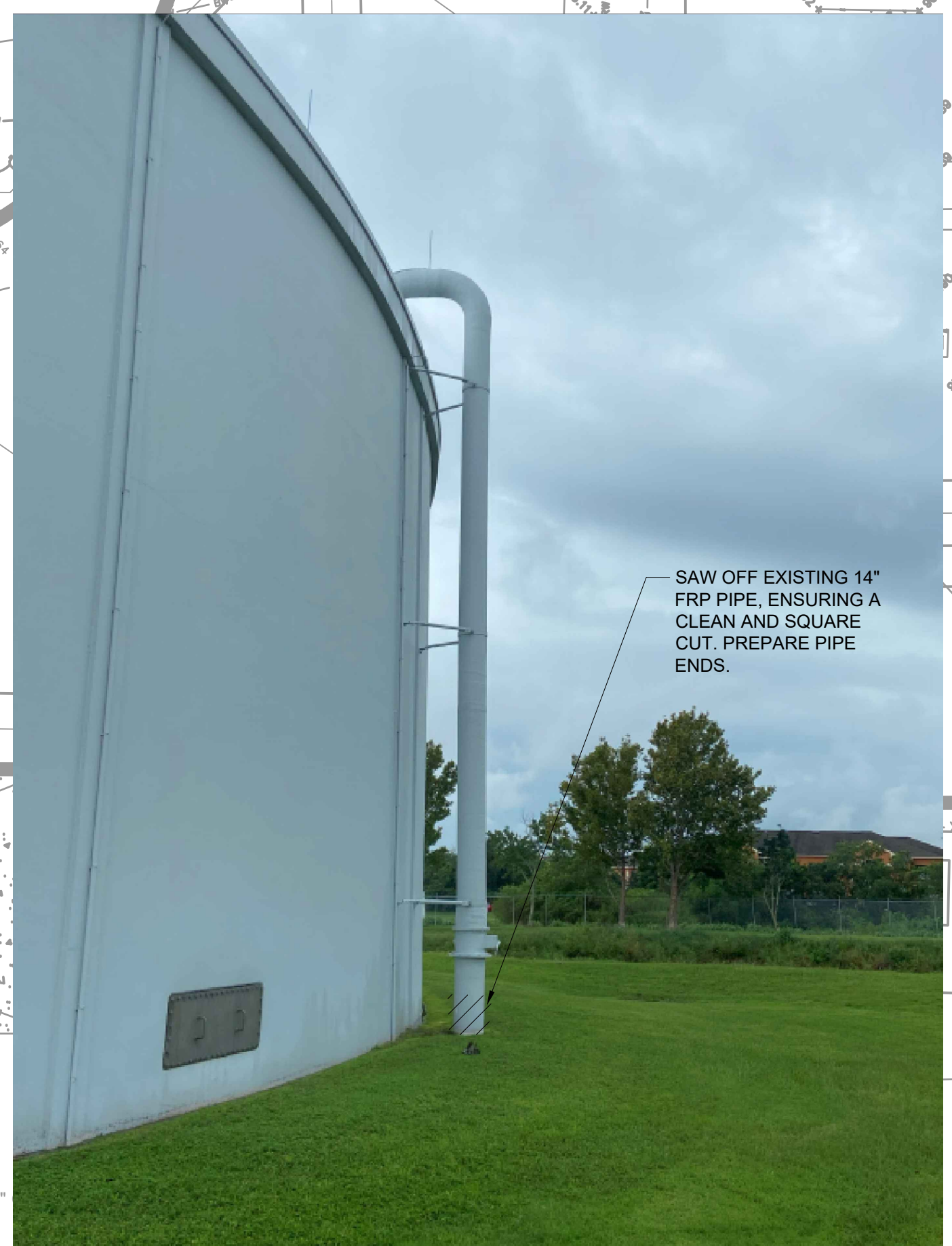
PHOTO 2 - ABOVE GROUND PIPING AT EQUALIZATION TANK
